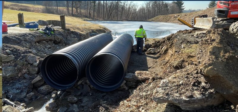
HIGH VOLUME STORM DRAINAGE
